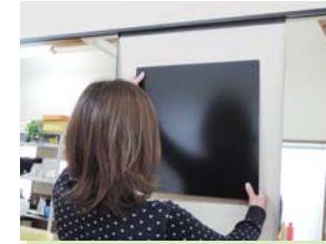
2.Mount a steel plate with screws and double-stick tape.
